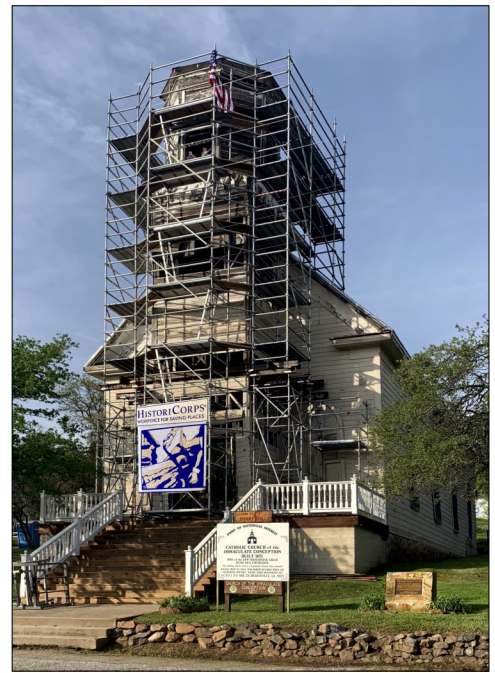
Scaffolding shows the ongoing progress of the Smartsville preservation project.
