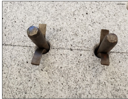
Paul explains the process as a fine crack is visible and the granite begins to split
