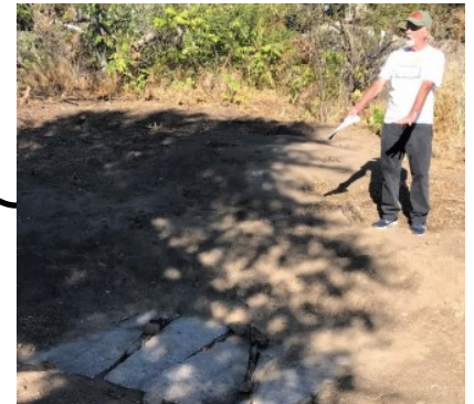
10. 19th-century storm drains/ granite culverts recently uncovered.
