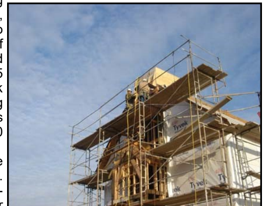
Building the bell tower and steeple
