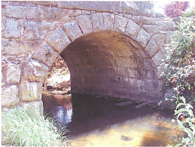
Clover Valley Bridge 2005
