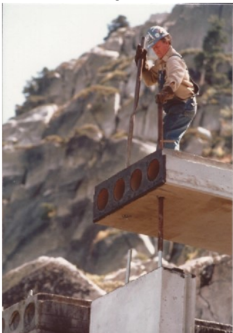
1984 Southern Pacific RR magazine photo showing George Schwartz working on construction of concrete snow sheds to replace wooden sheds.
