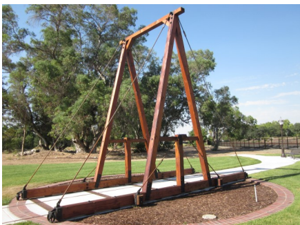
Rocklin Railroad Roundhouse engine turntable superstructure
